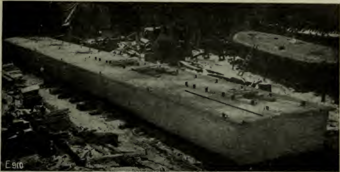
FIG. 5.—LARGE PONTOON READY FOR LAUNCHING.
